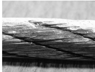
a. Excessive metal loss
